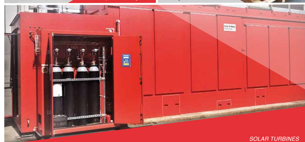
DATA CENTER FOUR Novec 1230 fire protection system
